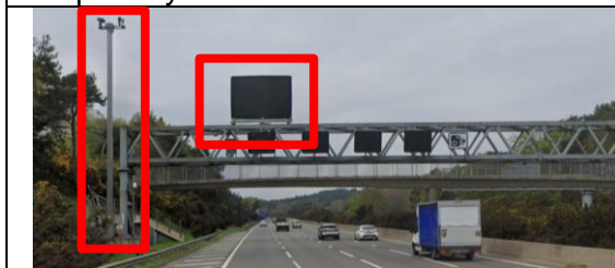
Figure 6A: Cantilever Gantry to be temporarily removed
