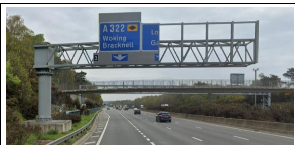
Figure 6B: Cantilever Gantry to be temporarily removed
